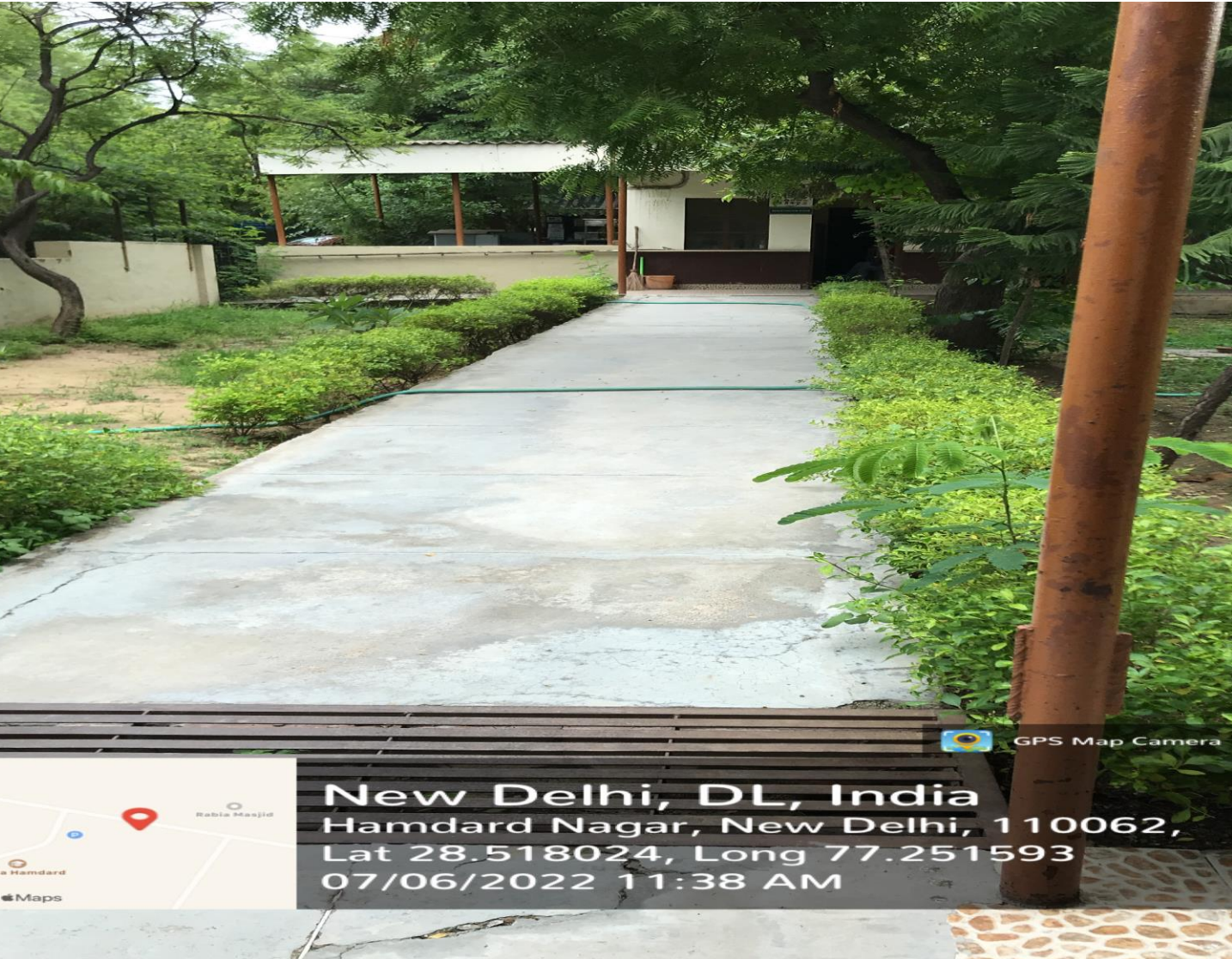
Ramp Rehabilitation Center JAMIA HAMDARD
