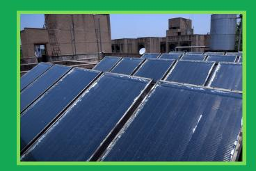
Solar Heating: The setup for using sunlight in order to heat up water in buildings in which the sun rays collectors are installed on roofs which pumps the heated fluid in a sealed circuit.
