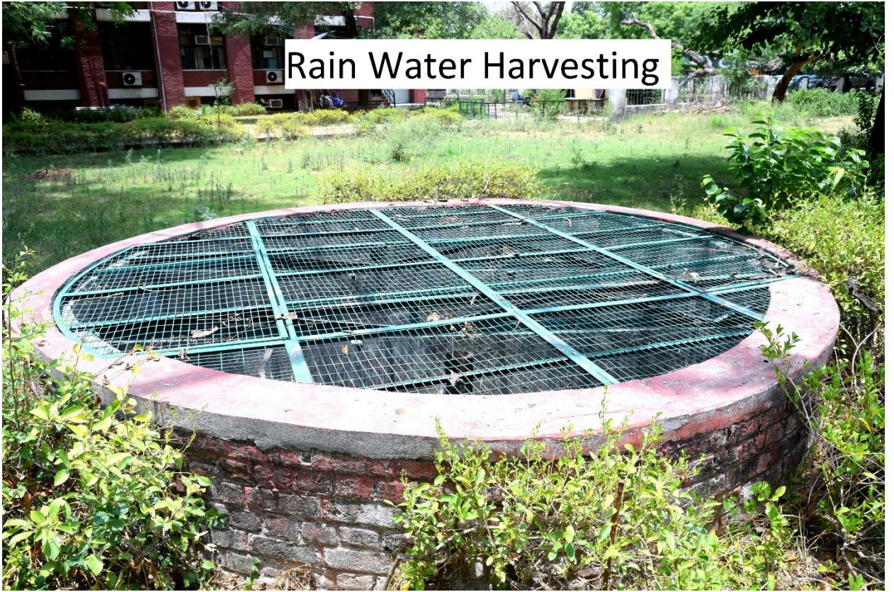
Rain Water Harvesting Well
