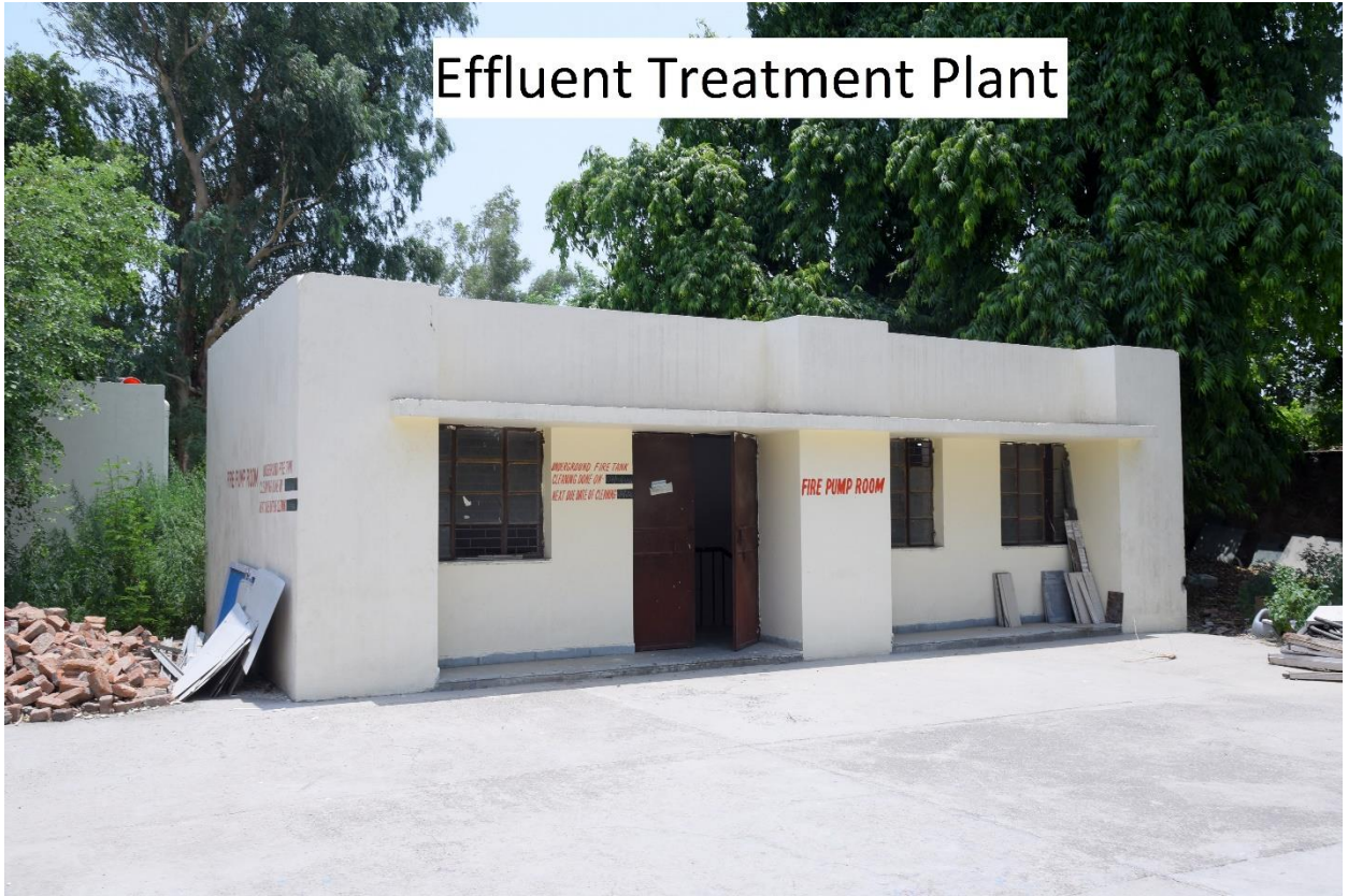
Effluent Treatment Plant
